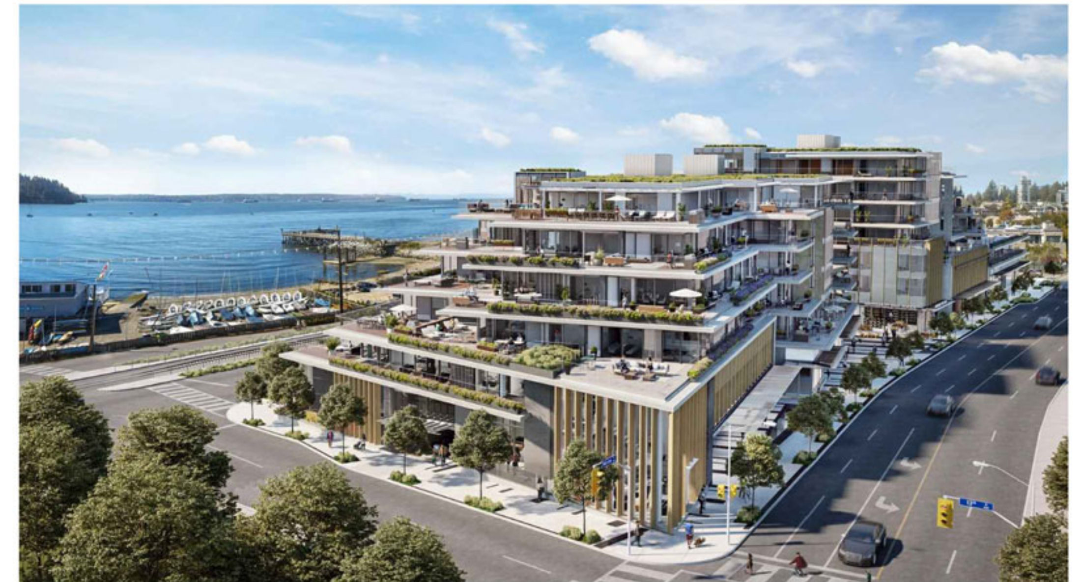
GROSVENOR AMBLESIDE MIXED-USE DEVELOPMENT - 13TH TO 14TH STREET BLOCK - SOUTH OF MARINE DRIVE
